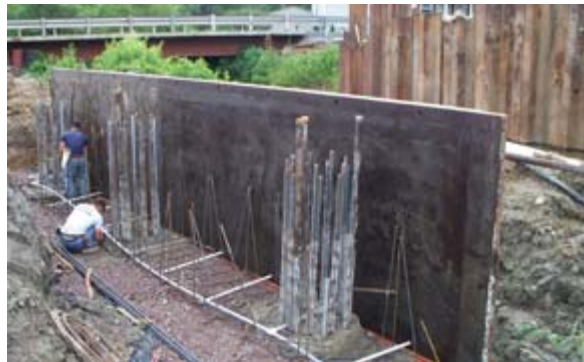
Reinforcement protruding from the tops of the three SCC caissons after completion.
