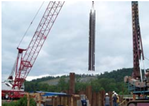
Reinforcement cage being lowered into place.
