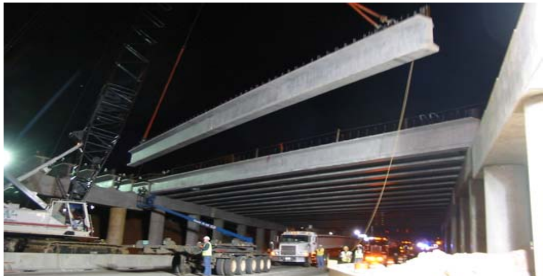
The use of high strength lightweight concrete reduced shipping weights.
