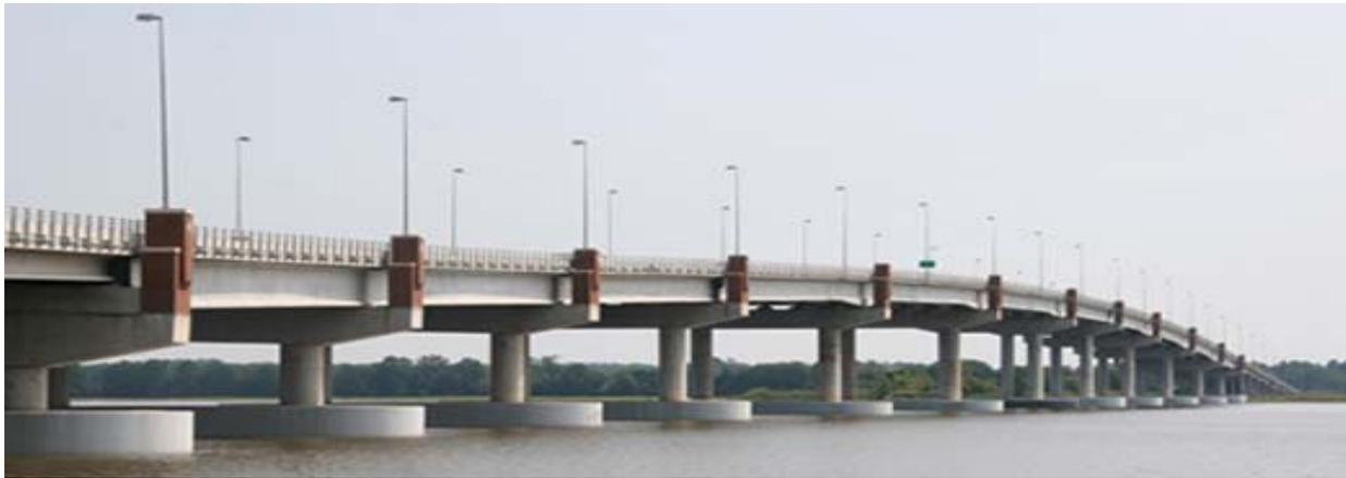
**High strength lightweight concrete was specified for the Route 33 Bridge over the Mattaponi River, VA.**
