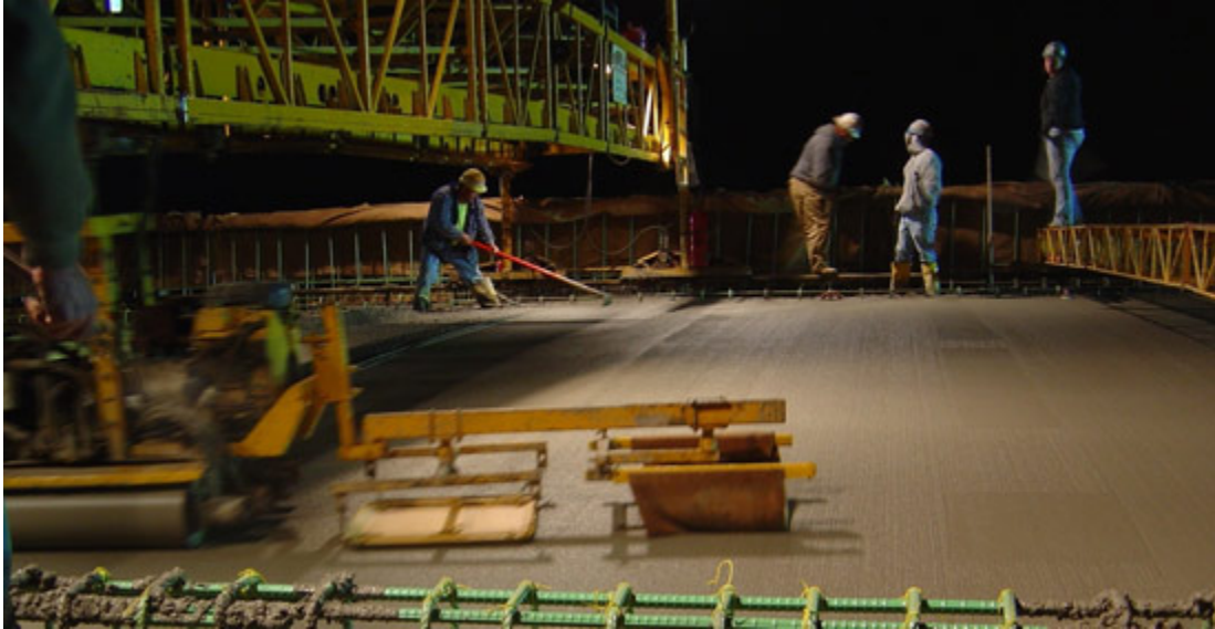
Casting an HPC bridge deck at night.
