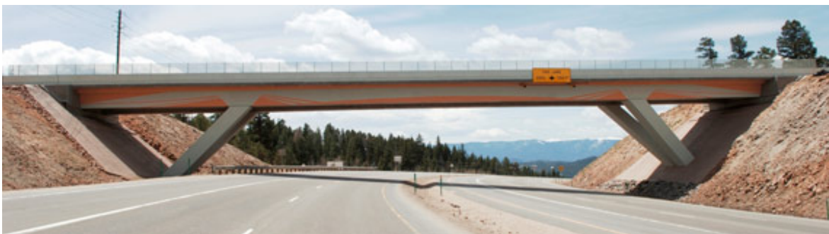
Richmond Hill Bridge, Conifer, CO. Photo: Steve Yip, CDOT
