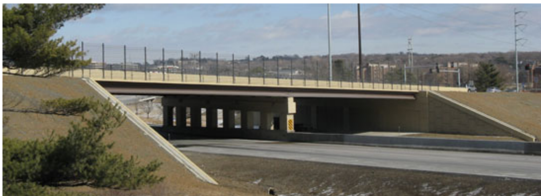
High strength concrete and 0.7-in. (17.8-mm) diameter strands were used in the precast, prestressed concrete beams.
