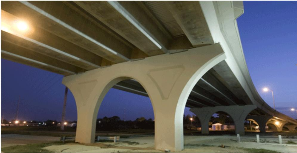
High strength concrete was used in the U-beams of the North Boulevard Bridge.
