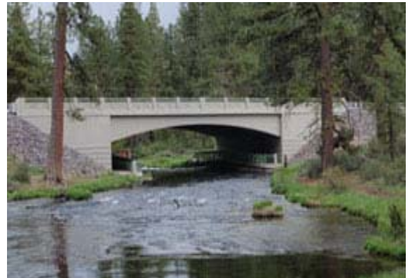
Replacement Collier's Promenade Bridge.
