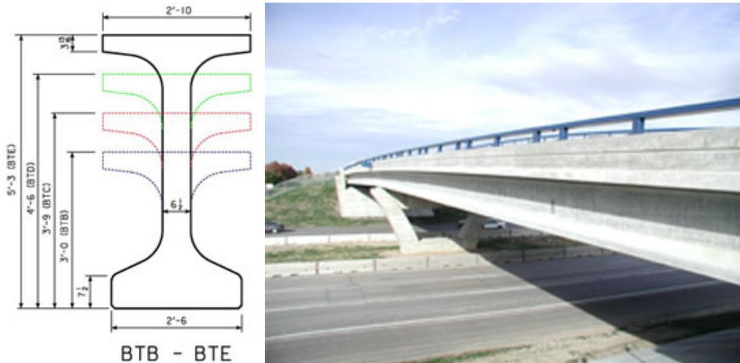
**Bulb-tee beam cross section and BT beam as installed.**
