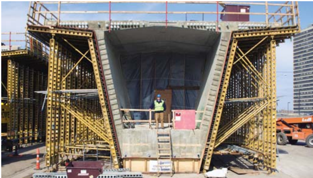
Precast concrete superstructure segment. Photo: Tim Davis, FIGG
