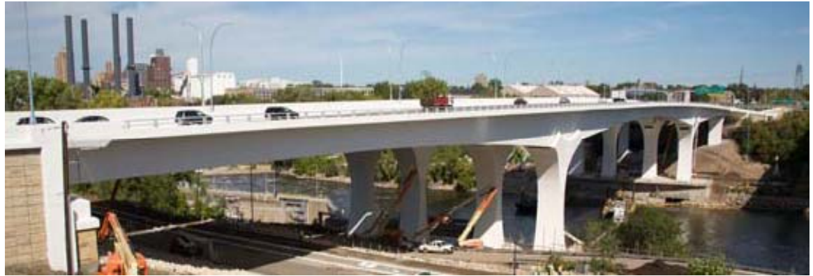
The new I-35W bridge across the Mississippi.
