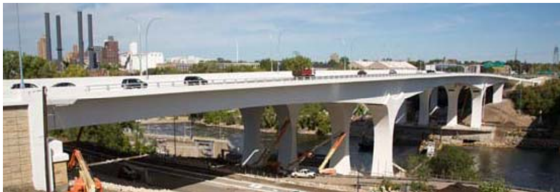
The new I-35W bridge across the Mississippi.
