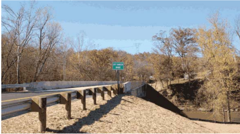
Sand-lightweight concrete was used to reduce the shipping and handling weight of the precast, prestressed concrete beams.
