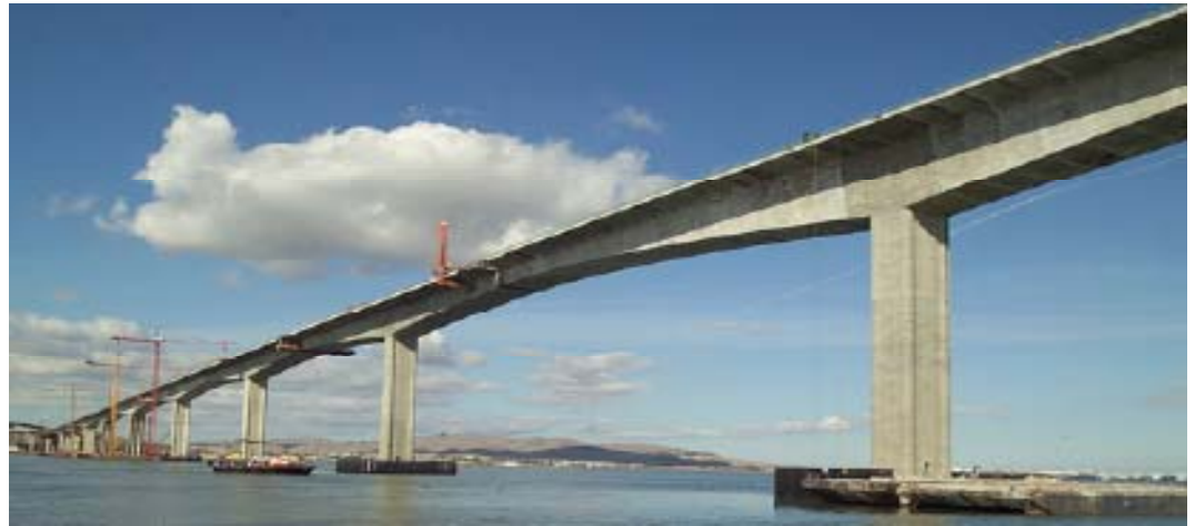
Lightweight high performance concrete was used for The cast-in-place superstructure segments.
