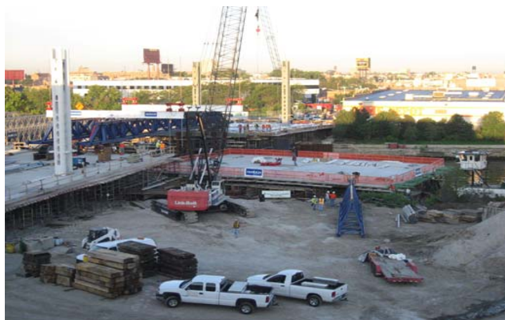
The center span was cast on barges and floated into position.
