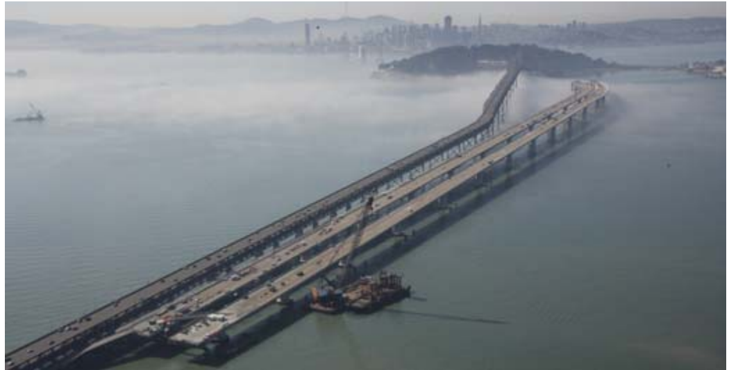
HPC was used in the Skyway to provide a 150-year service life.
