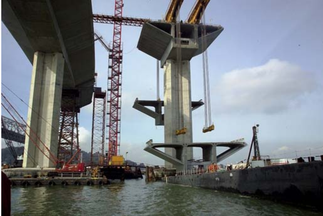
Erection of precast concrete segments from a barge.
